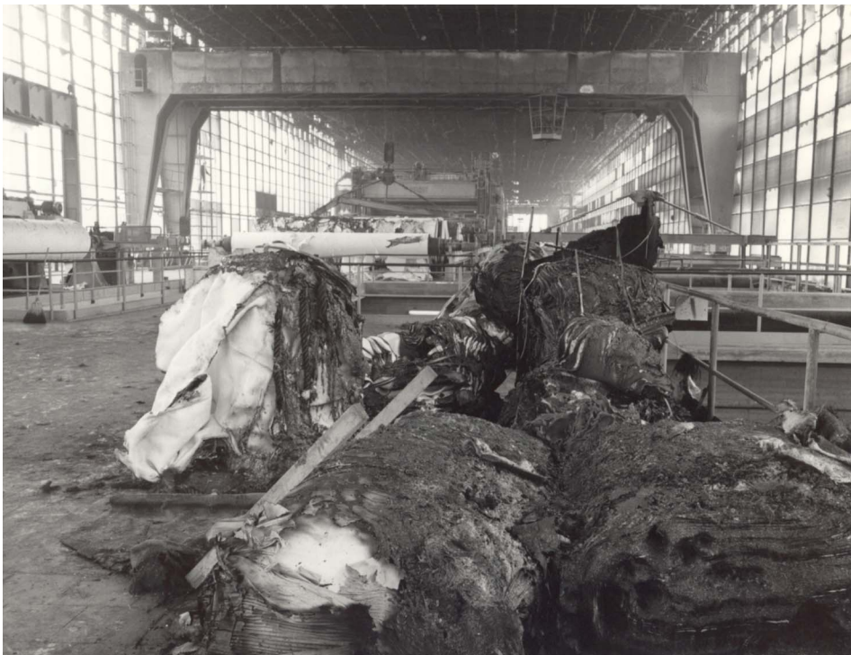
Figure 20. Photograph of the Burgo Paper Mill after the fire in 1974 [Burgo Paper Mill Archive, Mantua, Italy] (color figure available online).
