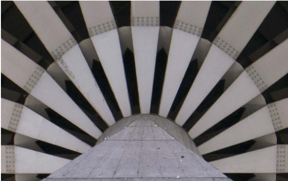
Figure 6. Detail of the bolted connection capital-beams [Manuel Cresciani's personal archive] (color figure available online).
