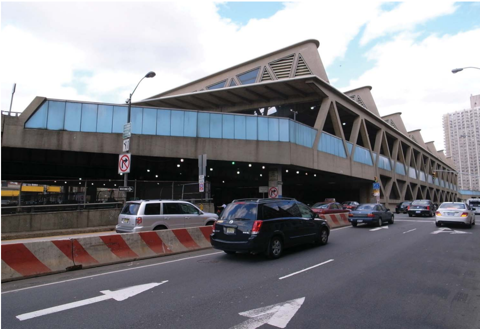
Figure 2. Photograph showing the two lattice beams and the structure of the roof [Manuel Cresciani's personal archive] (color figure available online).
