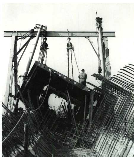
Figure 19. Diagram of a cross section (the reinforcement around the steel box, red in online files) and a photograph of the positioning of the hybrid connection between the support and the chain, the steel box [CSAC, Parma, Italy; Burgo, Mantua, Italy] (color figure available online).
