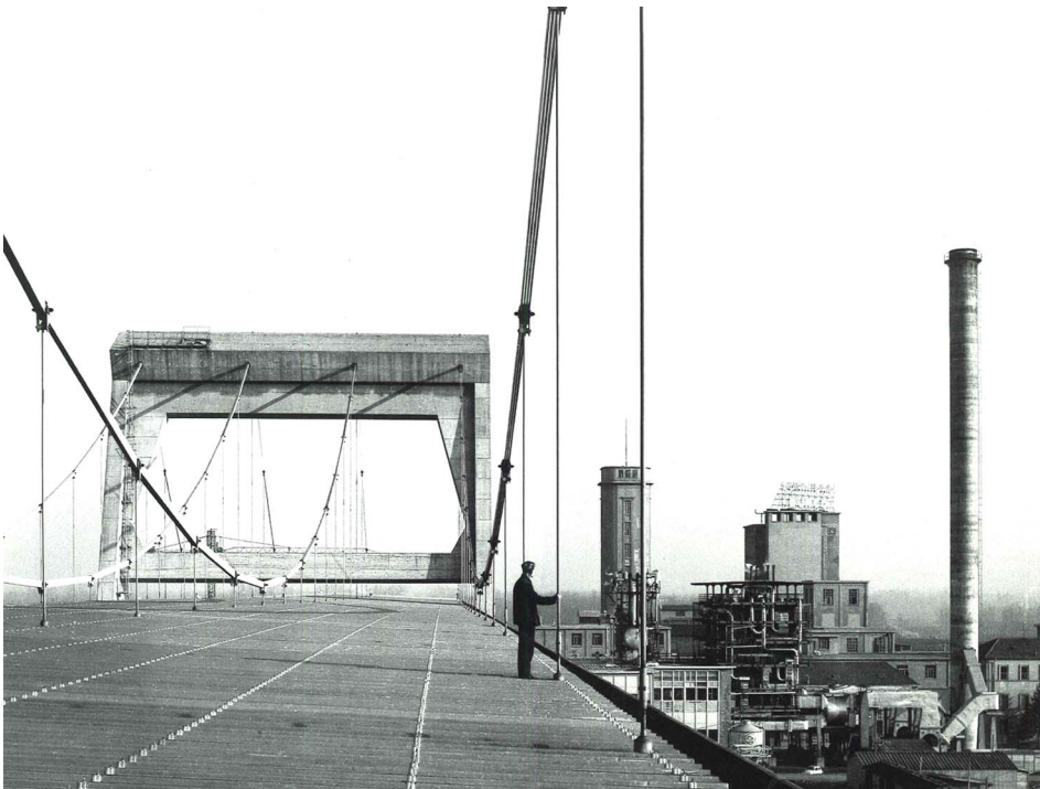
Figure 15. Photograph taken on the roof of the Burgo Paper Mill in 1961, Mantua [Burgo, Mantua, Italy] (color figure available online).
