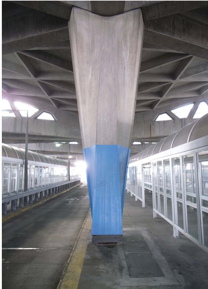
Figure 3. Photograph shows the variation in the profile of the central column [Manuel Cresciani's personal archive] (color figure available online).
